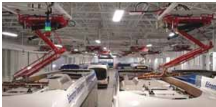
How electric buses would be recharged at the new facility. COURTESY PHOTO
